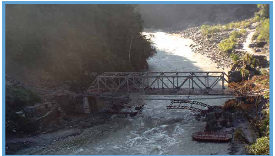
Road to Kimathanka, Bridge over Arun river
